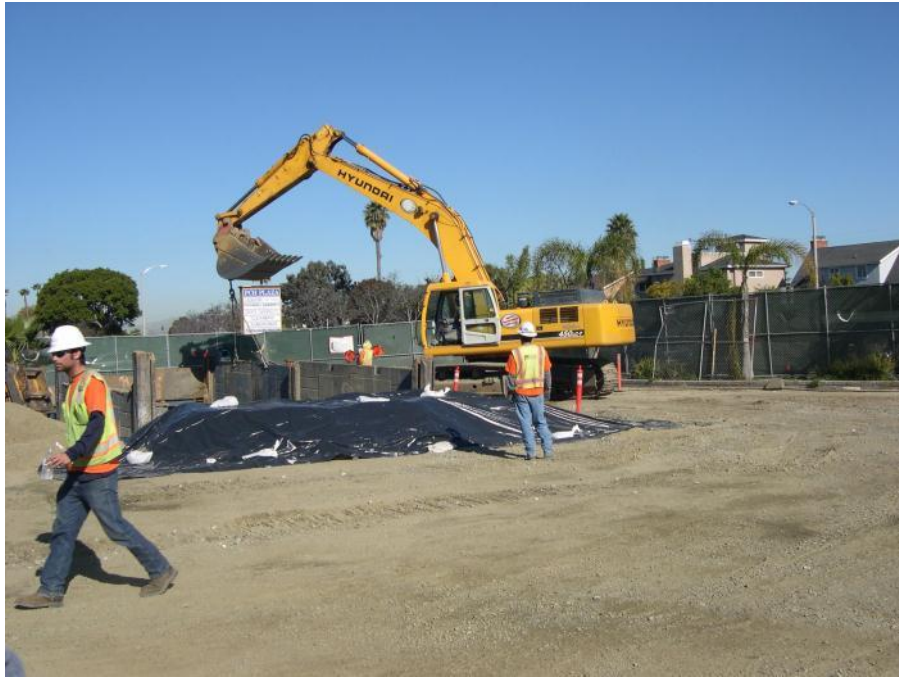
Excavation within cell
