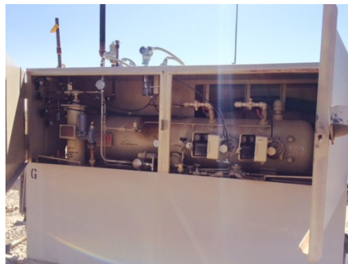
Figure 17-1 Picture of Equipment Building
