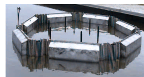
a. Steel Construction Boom
