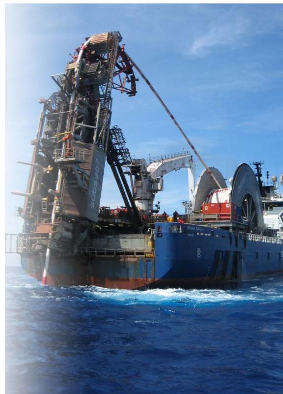
Figure 33: Marine Construction Vessel Installing Flowlines
