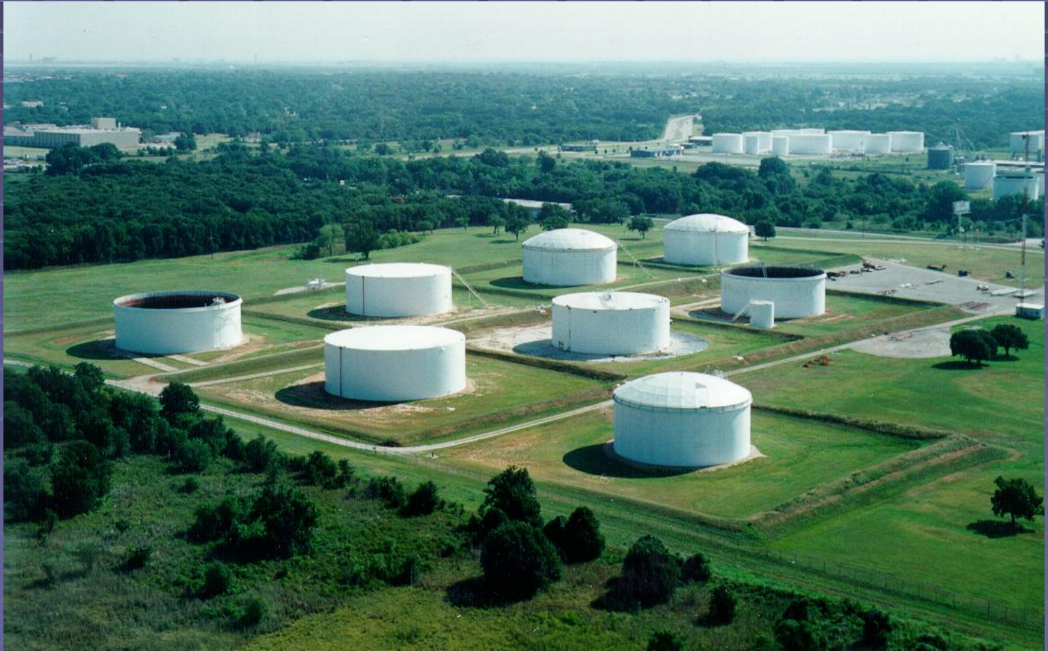
Field Constructed Tanks
